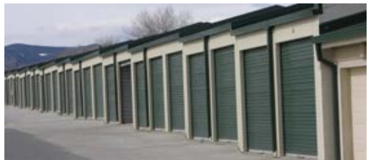
MINI STORAGE BUILDING WITH STEPS
