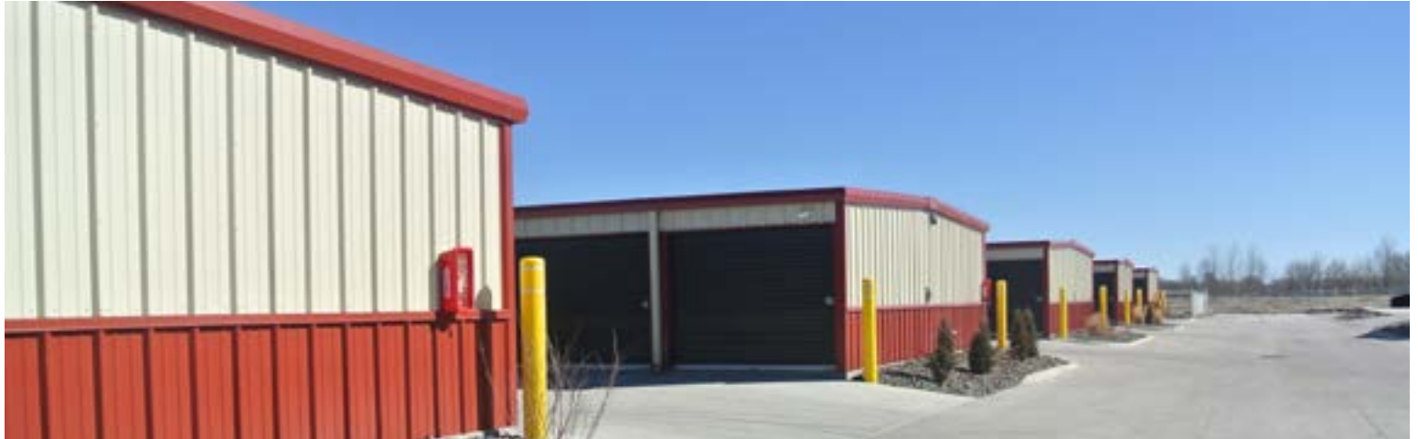
STANDARD .5:12 ROOF PITCH - GABLE
