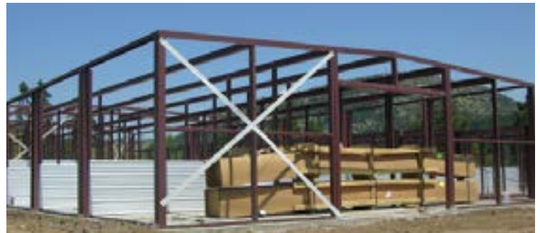
TEMPORARY BRACING
