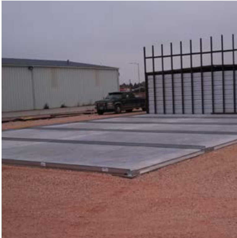
FOUNDATION WITH DOOR NOTCH AND BASE CLIP
